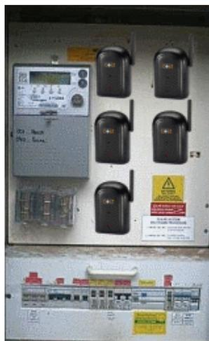
Note : There is no total household monitoring in this installation, as the client is uploading the monitoring data to an online web portal. Each of circuit's power data [except 5,6,7 as already included in P1/P2], will be fed into a virtual household total on the web portal. All circuits will show live, daily, monthly and annual data.
